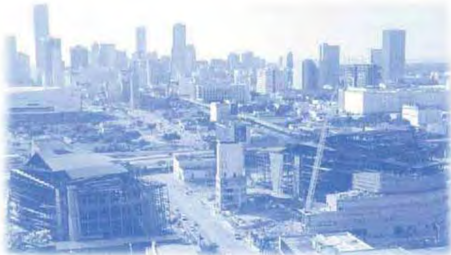
Performing Arts Center Construction Site
